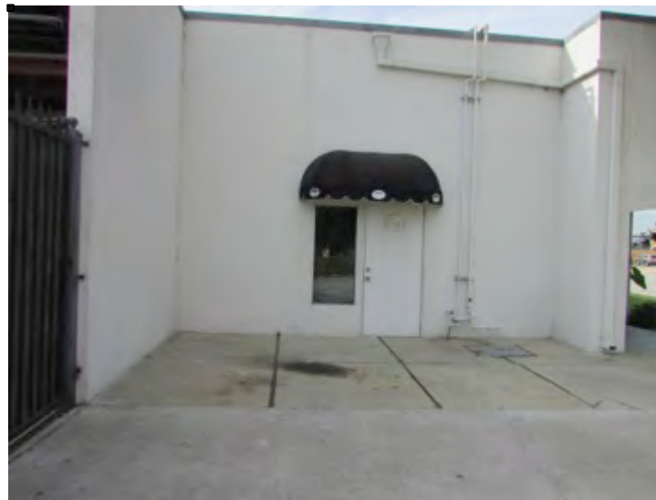
Figure 5. Overview to the west from locked and unattended gate blocking direct access to DE-APE
